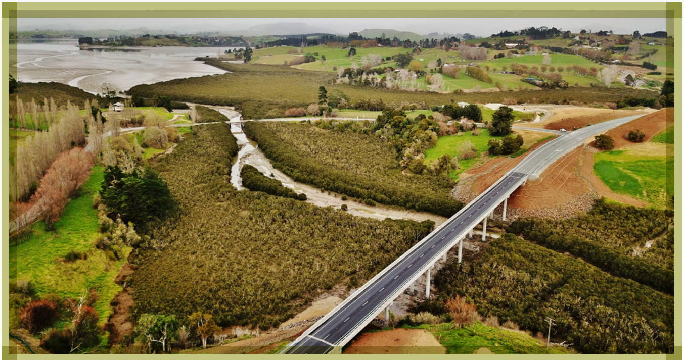
Piringatahi Bridge (Photo courtesy of Opus Consultants).
